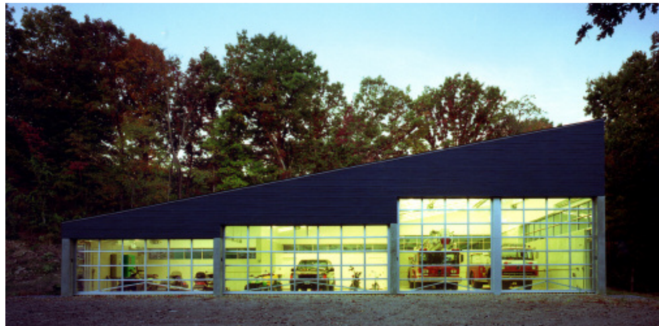
Pride of place in the Rusty Goat Garage belongs to the two fires engines, which dictate the shape of the structure. Martin Holub Architects (212) 787-7644 www.mharchitects.com
